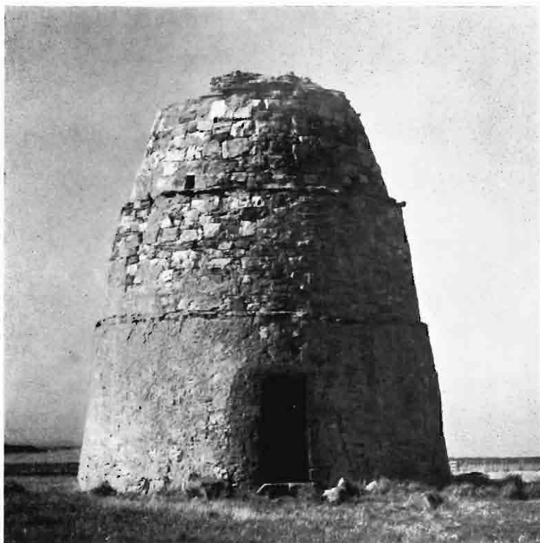
PLATE 1. Dovecote at Barnyards of Findlater, Banff-shire; the earliest type of dovecote in Britain; this one containing over 900 stone nestboxes (see page 22).
