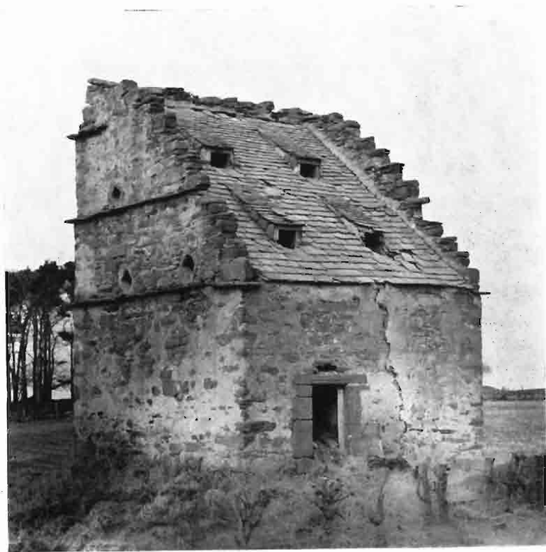
PLATE 2. Four-chambered dovecote at Leicheston, near Buckie, Banffshire: a typically Scottish design, but unusual with four compartments; this one containing about 450 nestboxes (see page 22).
