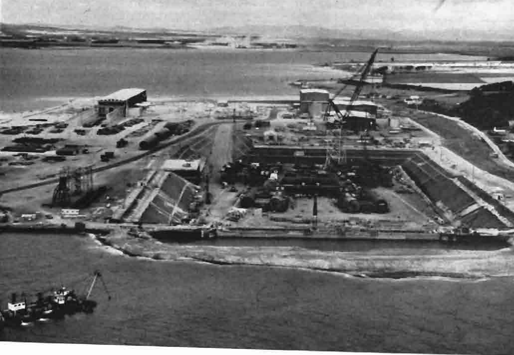
PLATE 1 (a). Oil-rig fabrication yard at Nigg Bay, Easter Ross, August 1973. The production platform for BP's Forties Field is being constructed in the graving dock (page 10). (b) The first North Sea oil pipeline coming ashore at Cruden Bay, Aberdeenshire from BP's Forties Field, May 1973 (page 8).
