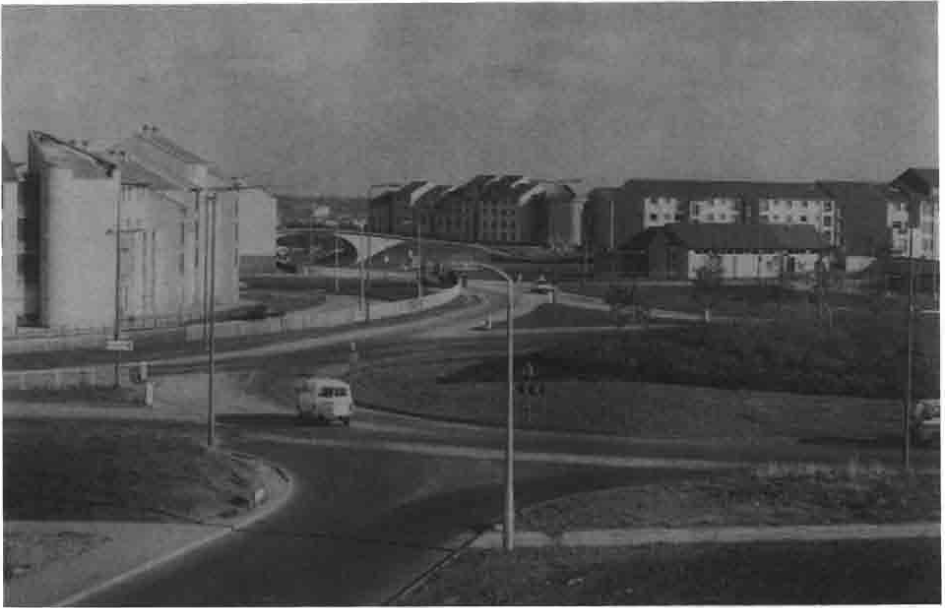
PLATE 4. Part of the Wester Hailes Estate, Edinburgh, where most houses do not have gardens.
