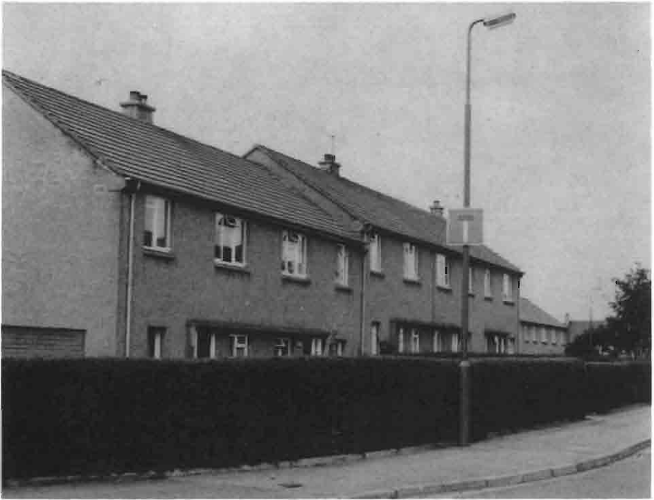
PLATE 1. Post-war council housing at Tranent with privet hedges important to nesting Blackbirds.
