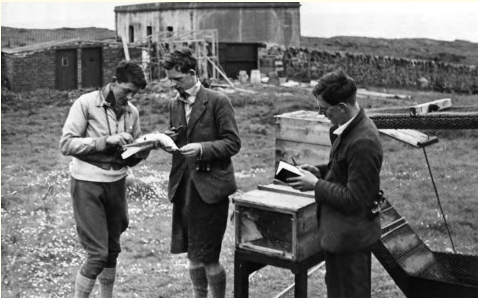
Plate 298. Frank Elder, Archie Bryson and Donald Watson (left to right) at the Low Trap in 1935, with the first ringing hut under construction in the background © SOC archive.
