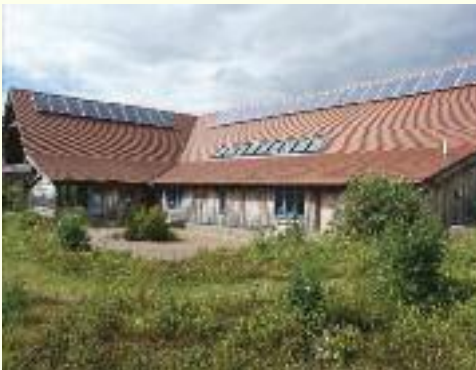
Plate 209. The 29 solar panels in place, June 2011. © Alan Fox
