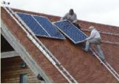
Plate 208. Installing the solar panels, Waterston House, June 2011. © Alan Fox
