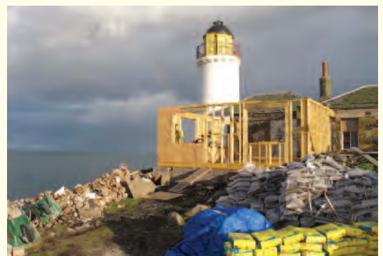
Plate 288. Low Light rebuild in progress. © Sofia Farinas
