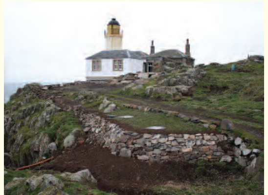
Plate 176. Observatory landscaping work, Isle of May, March 2014. © Mark Oksien
