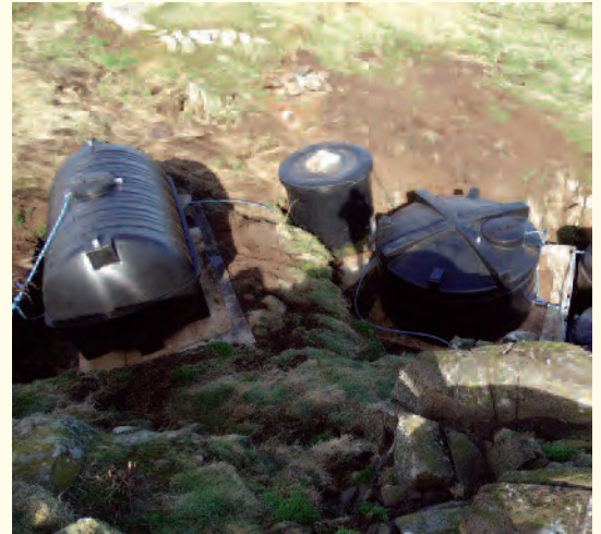
Plate 152. The new water storage tanks outside the Observatory, Isle of May, 2015. © Mark Oksien
