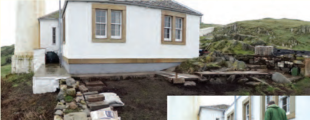
Plate 330. Observatory paths being built. © Mark Oksien
