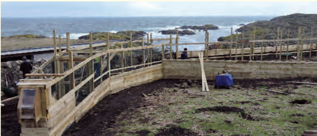
Plate 132. The new Bain Trap being constructed. © Iain English
