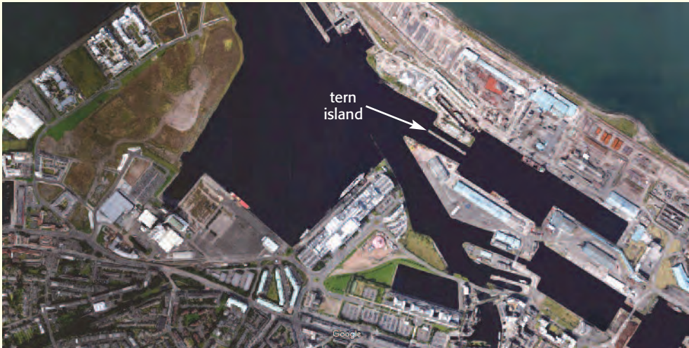
Plate 173. Leith Docks from the air. © 2018 Google
