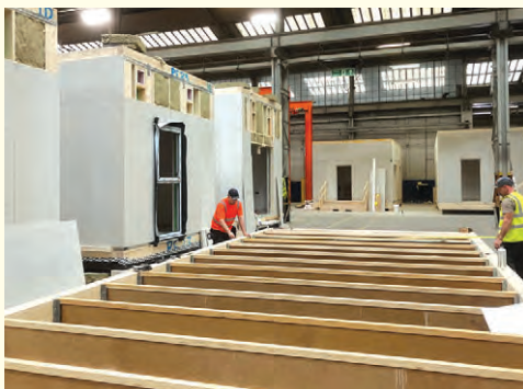
Plate 261. The modules under construction, Sheffield, South Yorkshire, 16 August 2022. © Ian Cowgill
